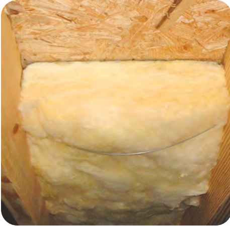
5. Batts are in good contact with subfloor
