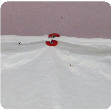
3. Seal seams of belly wrap
