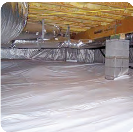
3. Spread out plastic as flat as possible
