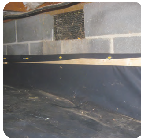
4. Extend plastic a minimum of 6" up walls, piers and columns
