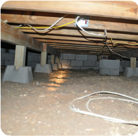
1. Clear out storage and debris
