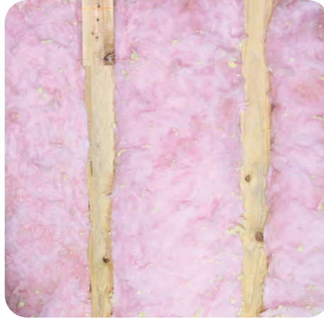
2. Cut batts for exact fit
