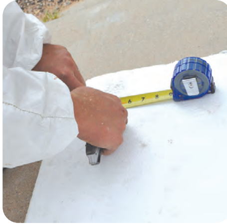
2. Cut blocking material to fit
