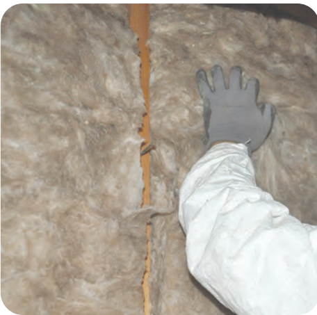
3. Install batts with minimal compression
