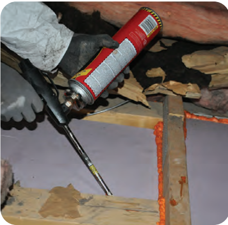
3. Ensure air sealing, if any, is completed
