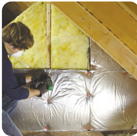
4. Install air-tight vapor-permeable backing material in contact with insulation
