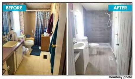
This before-and-after image is an example of a Home Rehabilitation Program project where a bathroom was transformed to be elderly-accessible, including a no-step shower, an elevated toilet and a grab bar.
