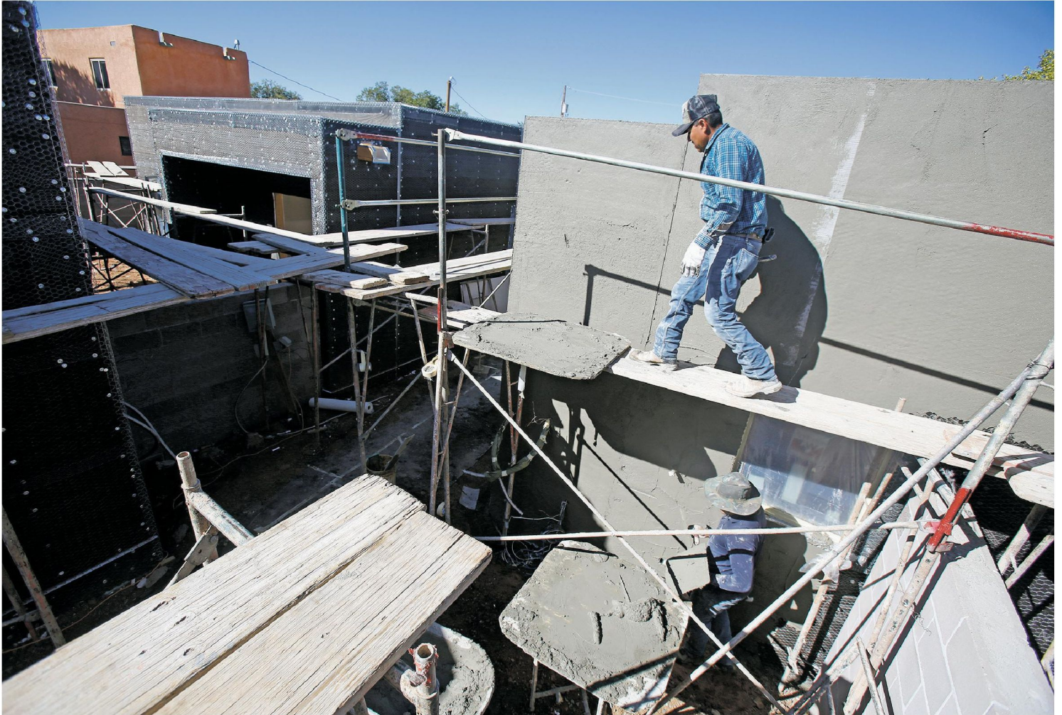
A crew with GMB Construction Inc. applies stucco to the Santa Fe Civic Housing Authority's Pacheco Street apartments Wednesday.
